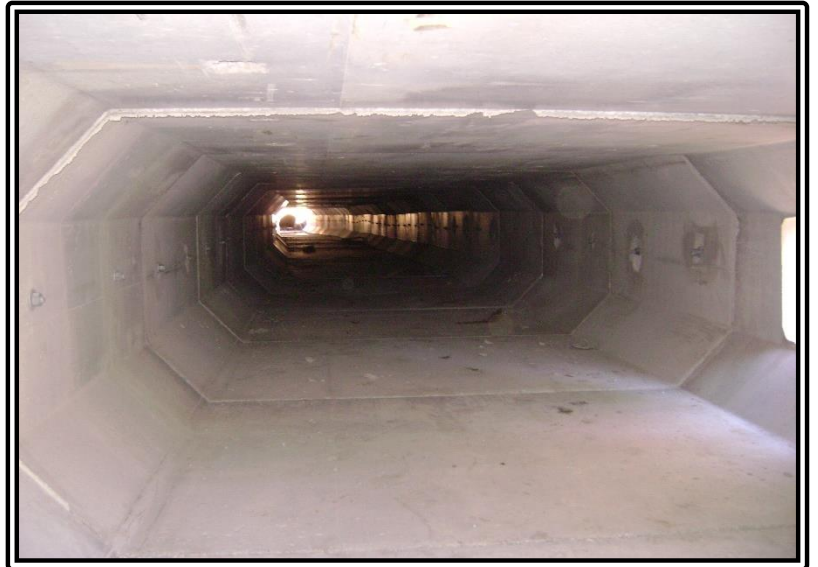
Mason Creek Culvert
