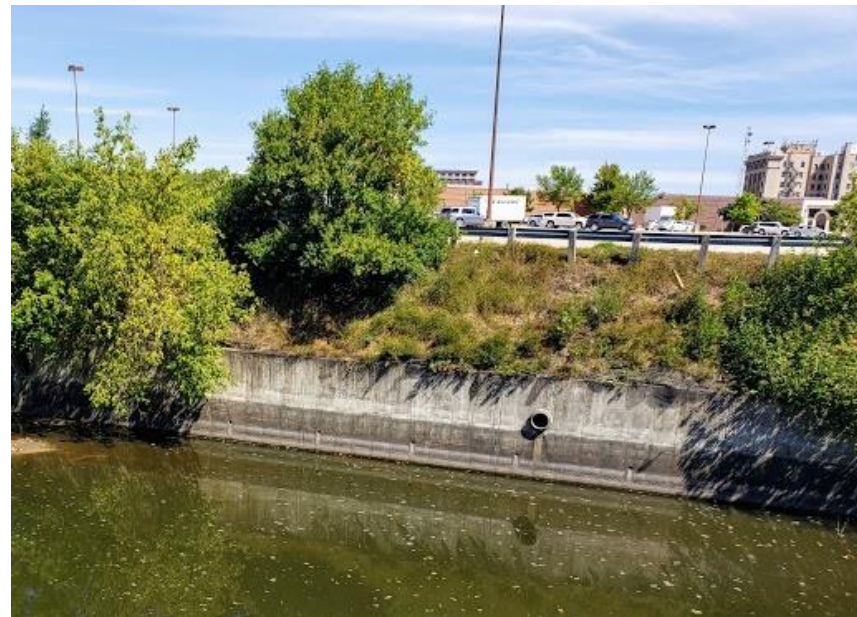
Storm sewer draining the Mall parking lot directly into Willow Creek
