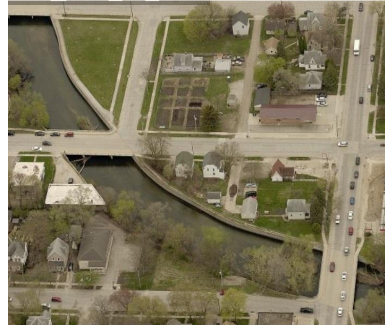
Concrete floodwall on the south side of Willow Creek, between the South Monroe Avenue and 2nd Street SW bridges (looking south)
