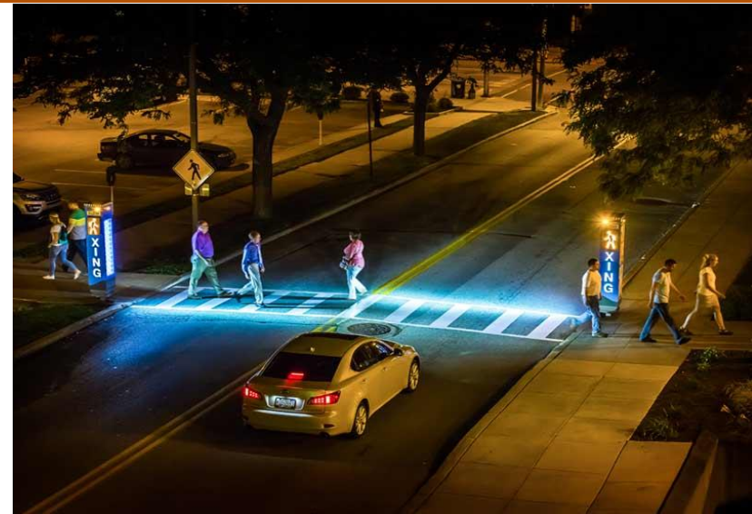
Example of a lighted pedestrian crosswalk (Howard Industries Prime Sign Program, http://www.primesignprogram.com/ped-crossing-signage.php )
