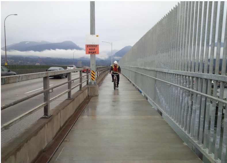
Protected bridge example
